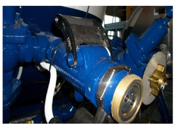
1.) Connect liquid spray fill and vapor equalizing lines ensuring a leak free seal.
